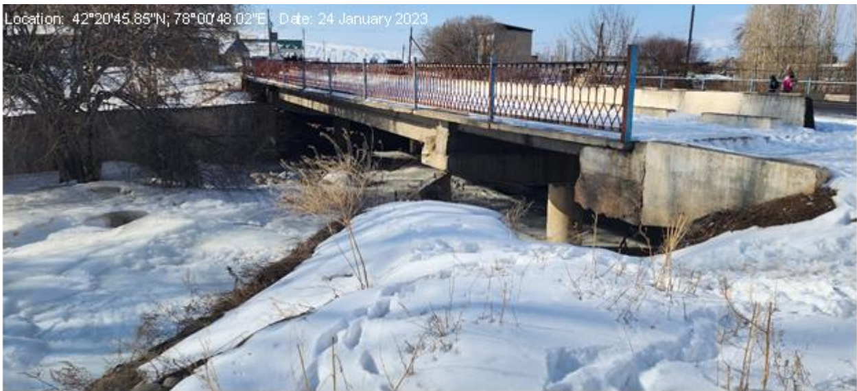
Figure 13: Existing bridge that will be replaced (KM 181+941)
