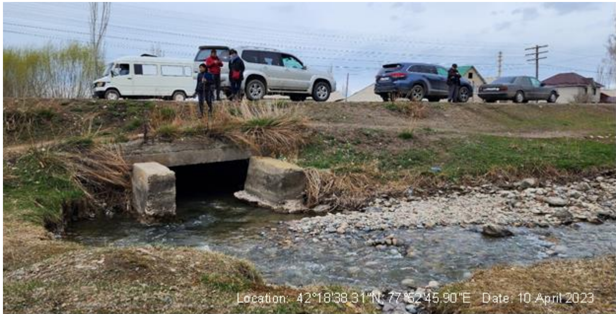
Figure 17: Existing culvert in Darkhan Village (KM 170+160).
