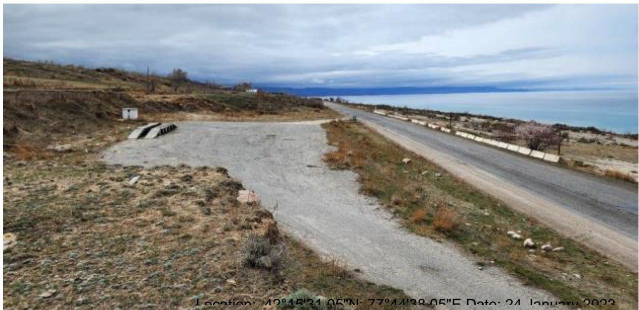
Figure 19: Existing parking/rest area where a new parking/rest area will be constructed between the villages of Ak Tarek and Zhenish (KM 157+438).
