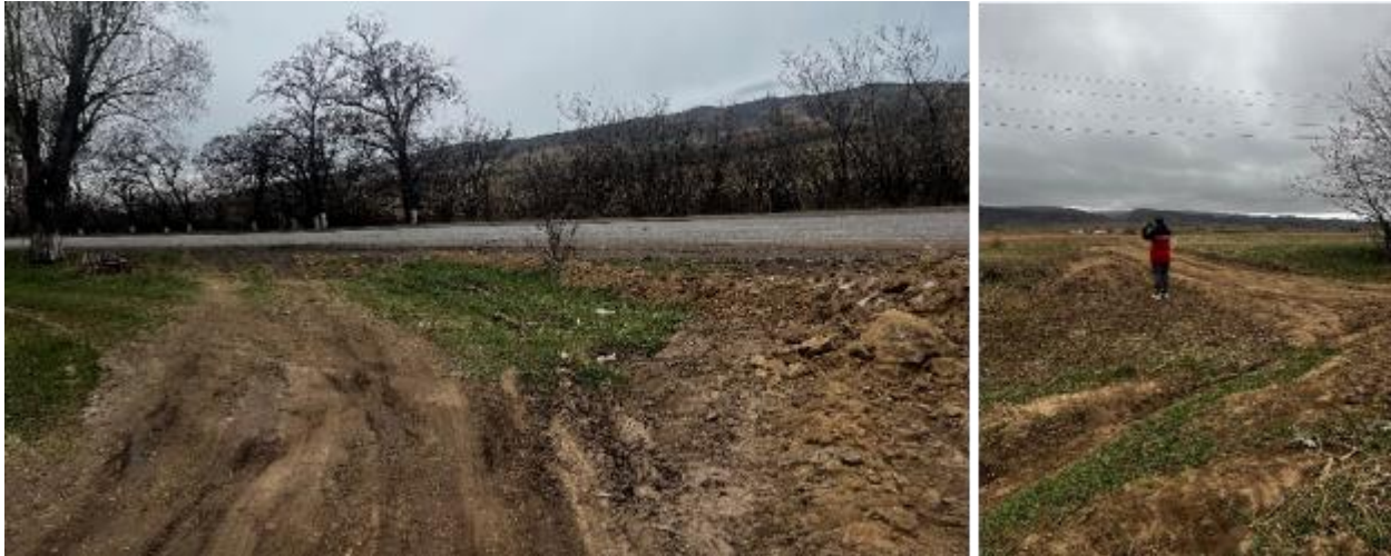
Figure 71: Section of the road affected by snow drift/flow in winter
