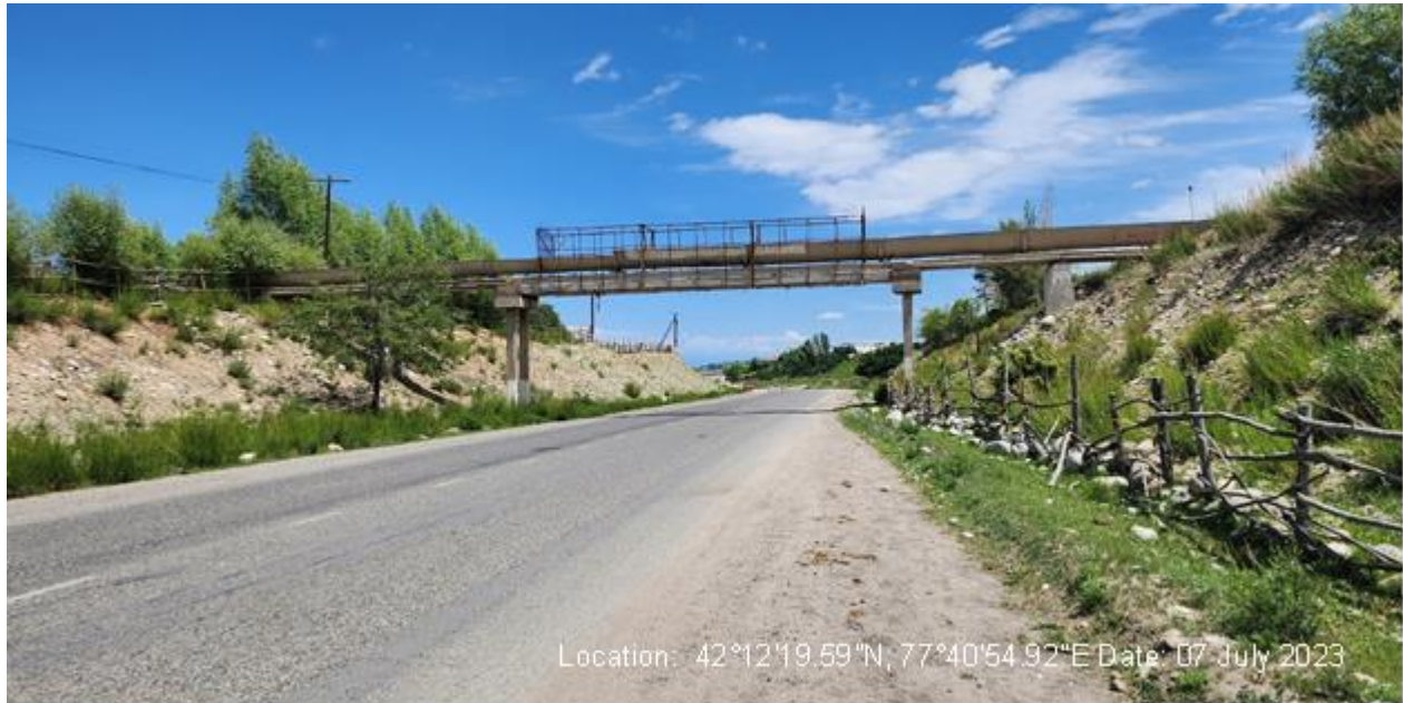
Figure 14: Existing aqueduct that will be replaced (KM 149+326.0).
