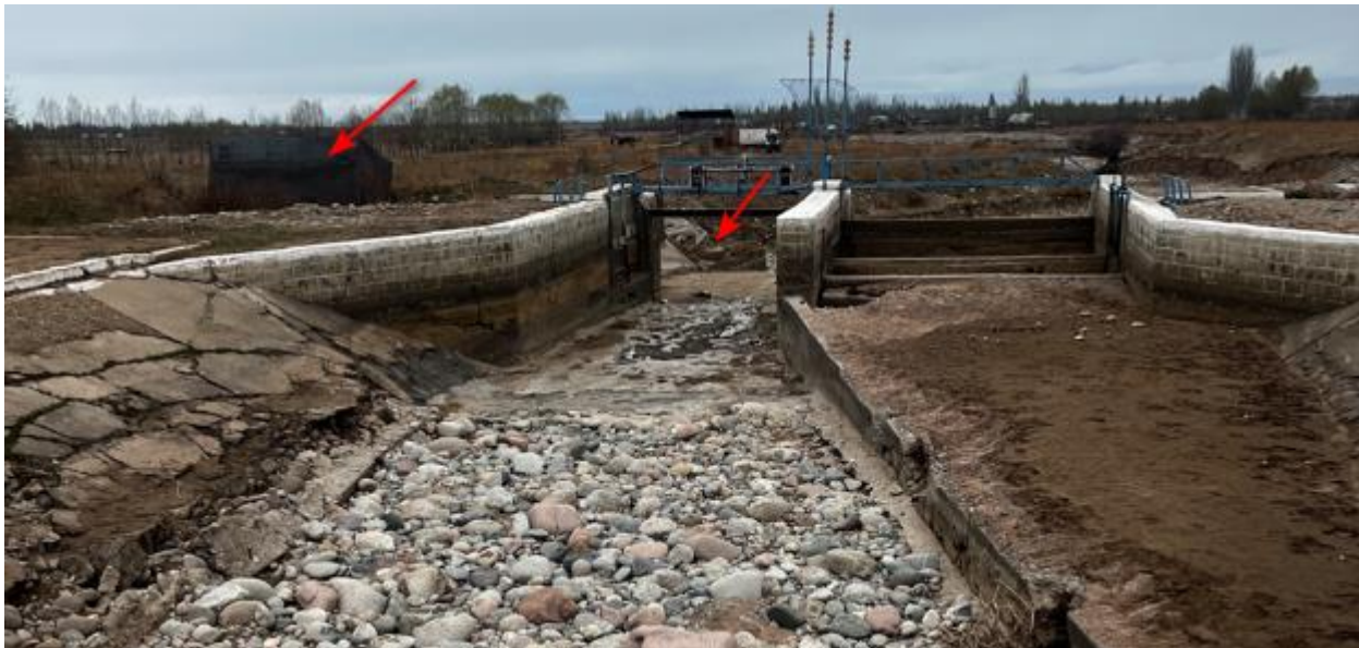
Figure 70: The dismantled hydraulic structure of the Jeti-Oguz Bridge
