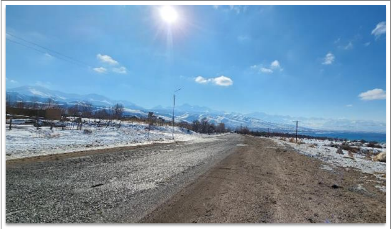
Figure E2: Existing road condition
